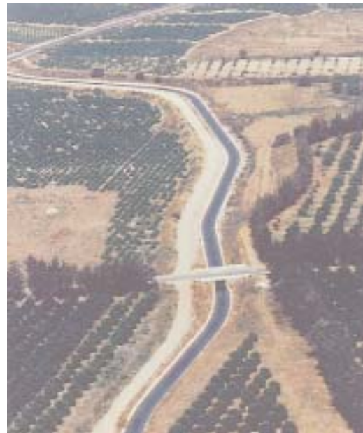
Paphos Irrigation Project. Central Canal (Photo: WDD Archive)
