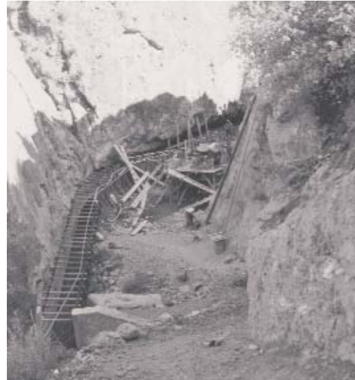
Construction of the foundations of the Trimiklini dam (Photo: PIO Archive)
