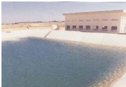
Southern Conveyor Project. Reservoir and pumping station for irrigation at Kokkinokhoría (Photo: WDD Archive)
