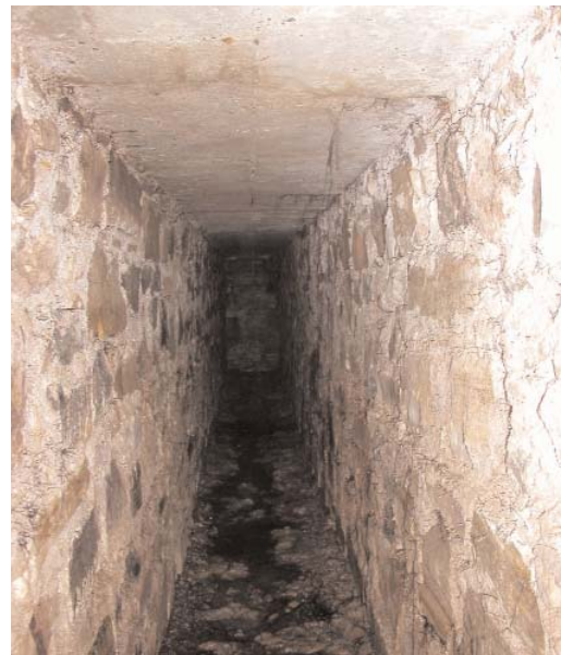
Underground stone built channel of the laoumi (Photo: WDD Archive)
