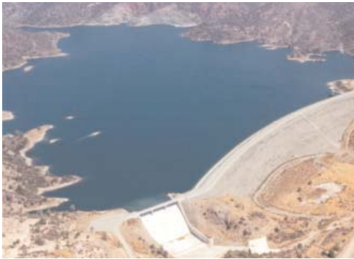
Vassilikos-Pendaskinos Project. Kalavassos dam (Photo: WDD Archive)
