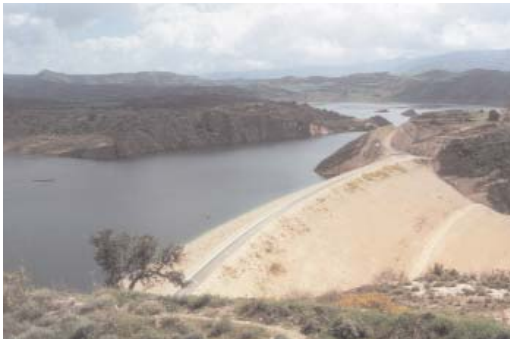
Khrysochou Irrigation Project. Evretou dam (Photo: WDD Archive)
