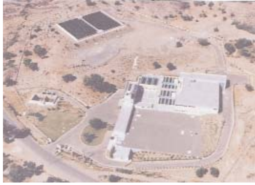
Vassilikos-Pendaskinos Project. Kornos Water Treatment Plant (Photo: WDD Archive)
