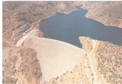
Lefkara dam (1973) (Photo: WDD Archive)
