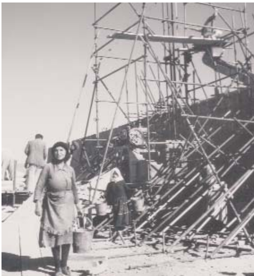
Construction of a concrete reservoir in Nicosia (Photo: PIO Archive)
