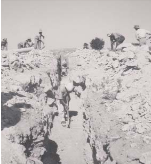
Placing of pipeline at Nicosia (Photo: PIO Archive)
