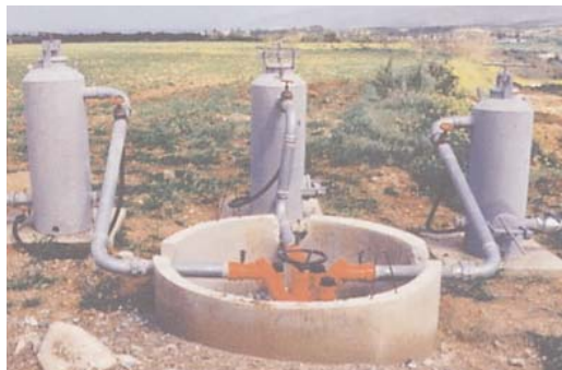
Khrysochou Irrigation Project. Triple outlet (Photo: WDD Archive)
