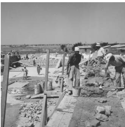
Construction of a reservoir in Famagusta (Photo: PIO Archive)
