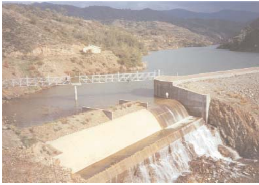
Argaka dam (1964) (Photo: WDD Archive)
