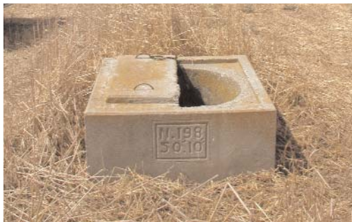
A view of a single well from a chain of wells for the water supply of the town of Larnaca (Photo: WDD Archive)
